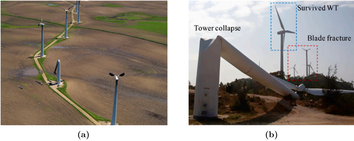
Fig. 1.1. Examples of wind-turbine failures caused by strong wind gusts in real-world environments: (a) Wind turbines at the Buffalo Ridge Wind Farm (Minnesota, USA, 2011) [4], (b) Wind turbines at a coastal wind farm (Shanwei, China, 2013) [5].
